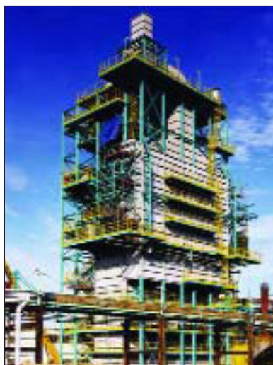
Ethylene Cracker Unit
