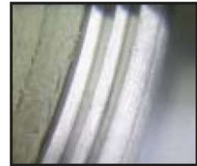
Profile of Change wire wound together beneath the facing.
